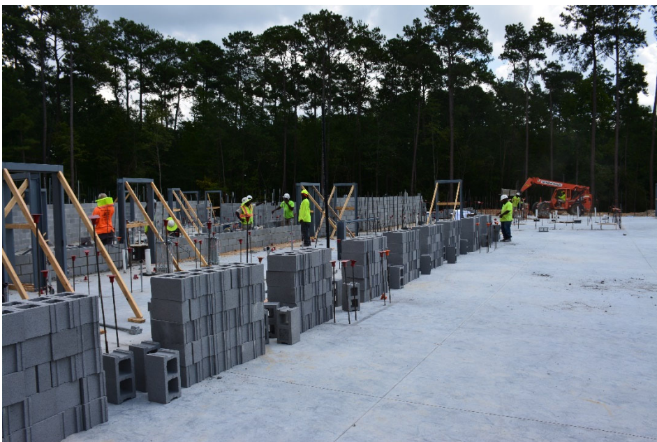
Class House 1 st floor masonry wall construction
