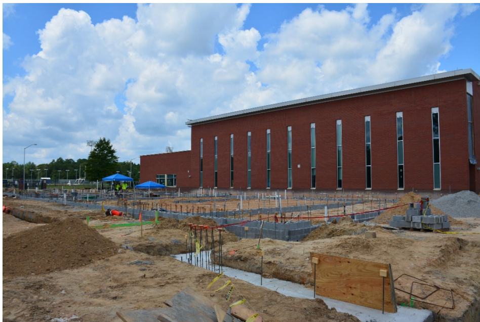
Multipurpose Addition footing and foundation placement
