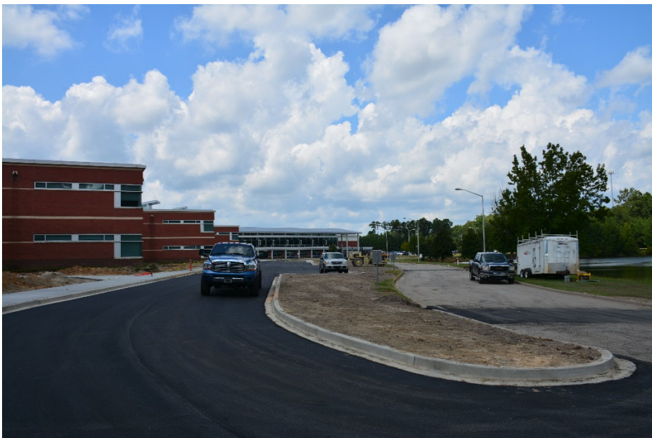
Base course pavement at temporary bus loop
