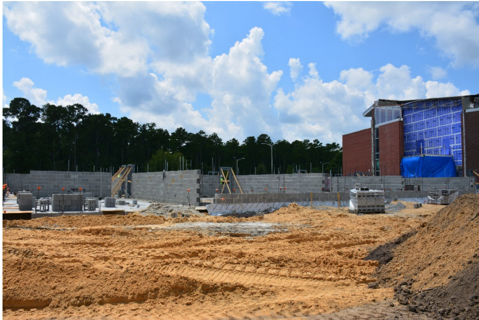
Class House 1 st floor masonry wall construction
